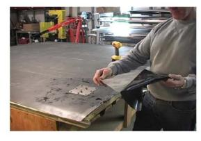
6. Apply target patch over base plate using proper mastics or welding installation techniques (varies with type of roofing material) so as to create a water tight patch.
