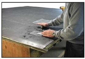
7. The threaded studs are now the only part of the base plate exposed. NOTE: Due to the sealer applied around the studs there may be "bleed out" at the openings.
