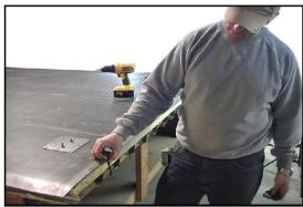
Be sure the fasteners are long enough to penetrate a minimum of 0.5" into the deck (not including the tip of the screw).
