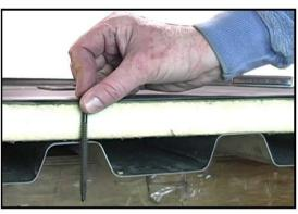
3. Align the base plate with the Support allowing for enough distance to connect the Polar Bear Connector Arm to the Support and ensuring that the Support will not interfere with the target patch. Use 8 fasteners per base plate.
