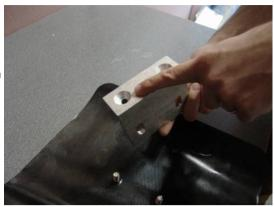
9. Place the countersunk holes over the studs and fasten the L-foot in place with the included neoprene bonded washers and stainless nuts.
