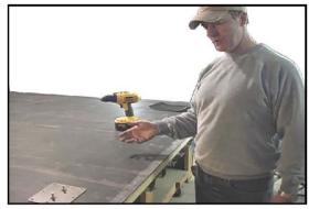
2. Use the right fastener for the roof and deck you are working with. Eco-Fasten has tested fasteners for use with steel and wood decks. Those test results are available on the Eco-Fasten website <a href="http://www.eco-fasten.com/pdf/ASG-Pull-Test-Report.pdf">http://www.eco-fasten.com/pdf/ASG-Pull-Test-Report.pdf</a>. Fasteners for concrete and other decks will need to be determined by the project engineer.
