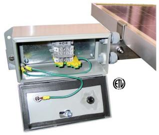
To securely mount the PTWB to the PV array racking structure, begin by determining a desirable location that will be easily accessible. The PTWB is designed to be mounted directly on the mounting rail. Use the supplied 3/8'' bolt on the mounting bar to attach the PTWB in the channel of the rail by sliding the bolt head in from the end.
