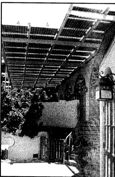
The solar panels shade a tiled deck outside the Libitzky's ballroom.
