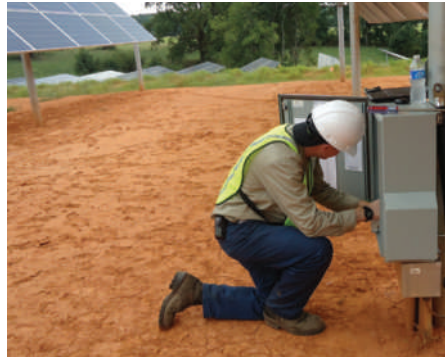
groSolar project and construction expertise and exceptionally high quality standards
