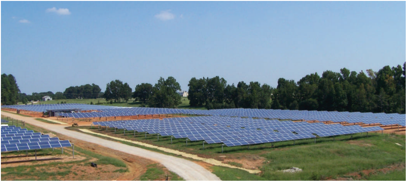
Advanced tracking technology from RayTracker GC is used to maximize output
