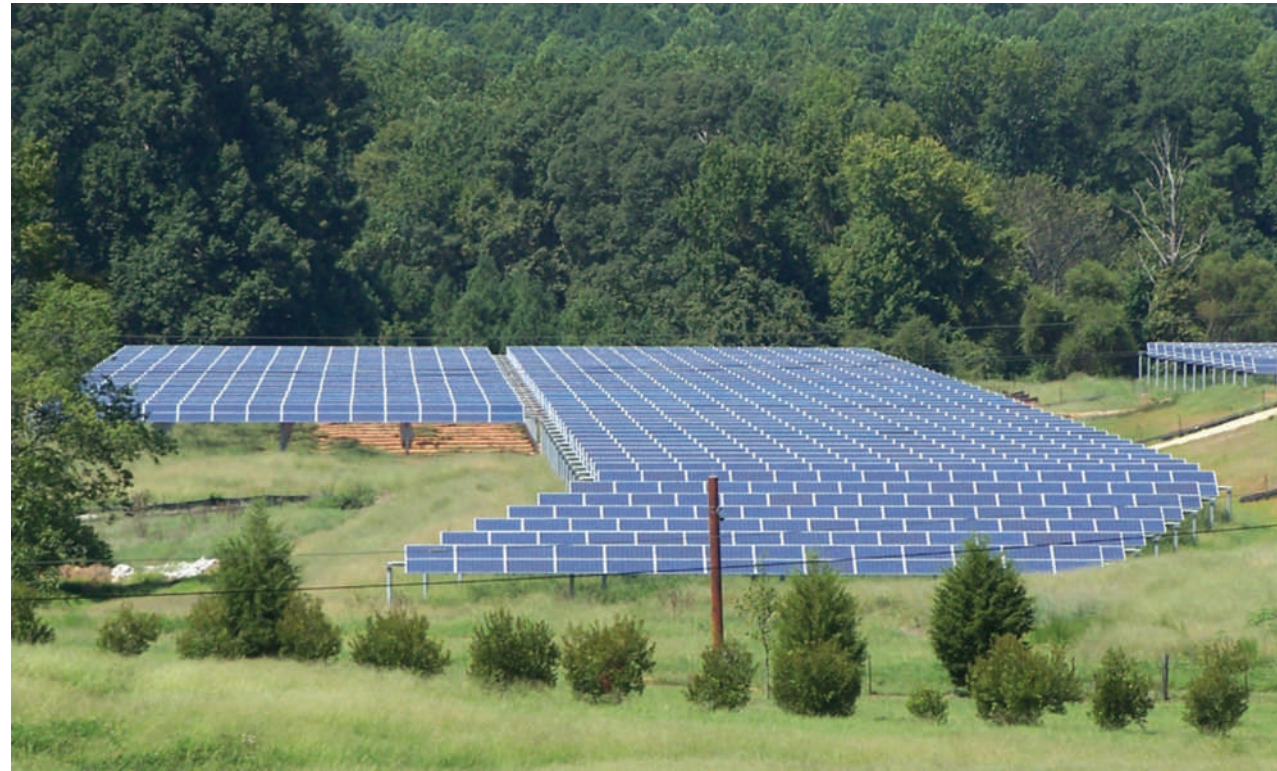
groSolar matches the natural environment with a terraced site design and RayTracker GC
