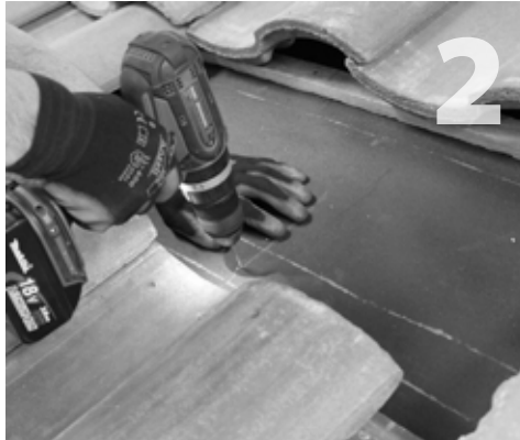
2 Rest the base plate (item 1) over center of rafter and mark center of holes. Drill two 7/32" pilot holes and fill with sealant compatible with roofing material.
