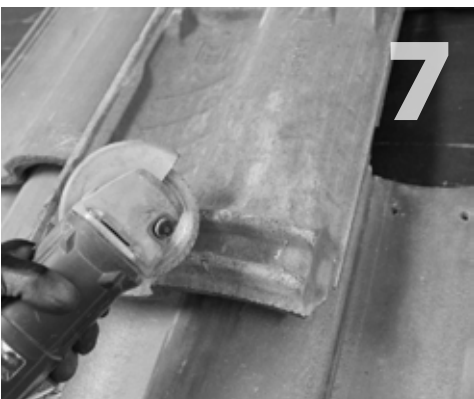
7 Replace the tile above the hook. If necessary, notch the bottom of the tile to make space for the raised hook.
