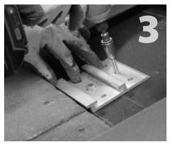
Drive lag screws into rafter through the two holes to a solid, snug fit. DO NOT over tighten lag screws, this may compromise their holding strength.
