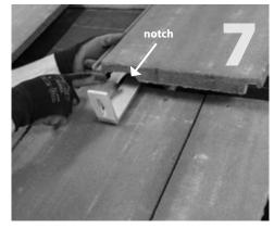
Replace the tile above the hook. If necessary, notch the bottom of the tile to make space for the raised hook.
