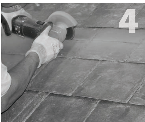
Using a cutoff wheel in a grinder, score the slate above the mounting area at 4 inches above the center of the QBase location. In step 5, you will remove the slate below the score line, which will allow you to slide the flashing up under the remaining slate in step 10.
