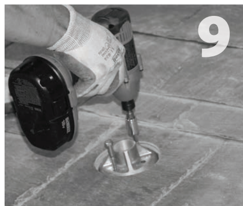
Prior to mounting to the roof, seat the grade-8 cap screw (item 1) through bottom of QBase. Secure the QBase to the rafter with (2) 5/16" lag screws (item 3) and tighten to a snug fit.
