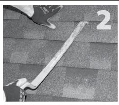
Carefully lift composition roof shingle with roofing bar, just above placement of Quick Mount.
