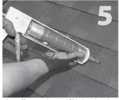
Clean off any sawdust, and fill hole with sealant compatible with roof material.
