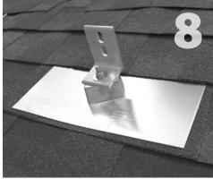
Using the rack kit hardware, secure the rack of your choice. Tighten to 13 foot pounds.
