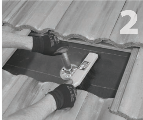
Clean away dust and debris around QBase.
