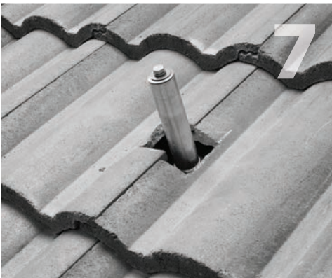
With a diamond blade on a grinder or skill-saw, cut tile to allow post to pass through. Place cut tile back in position. Insert post (item 3) and tighten into place.
