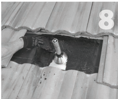
After first layer of cement is dry apply second layer over reinforcing fabric to finish waterproofing of subflashing.
