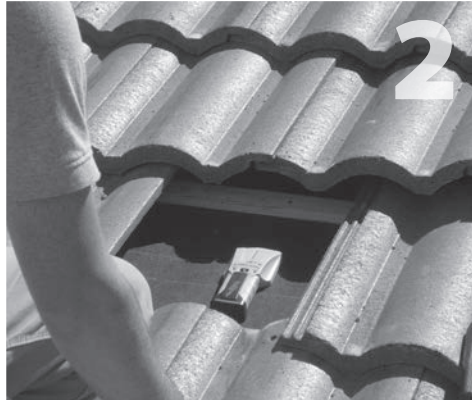
Locate and mark center of rafter. Clean felt paper with hand broom.
